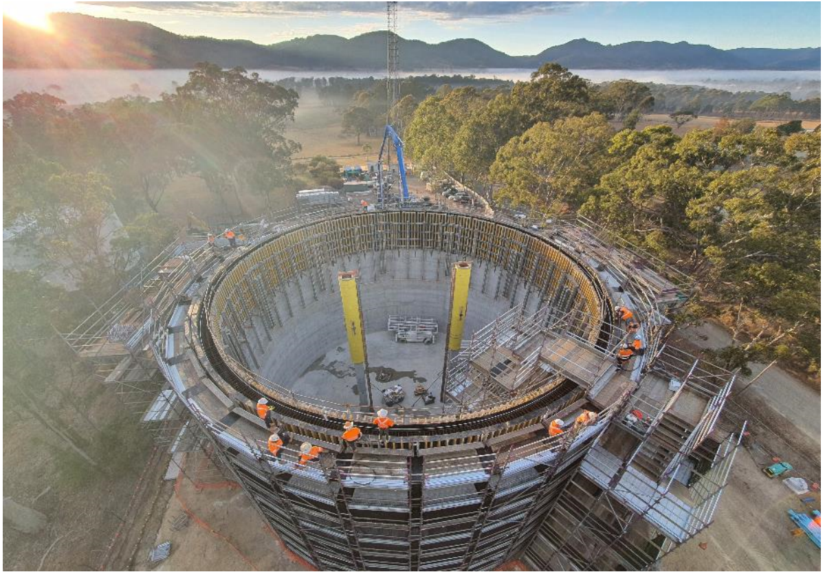
Figure 5: Construction of concrete reservoir in Gloucester Water Supply System
