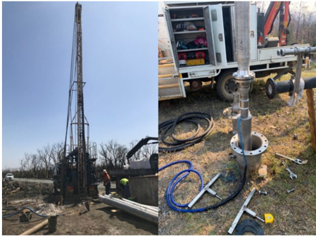
Figure 2: Installation of new bores at NABIAC Water Supply System
