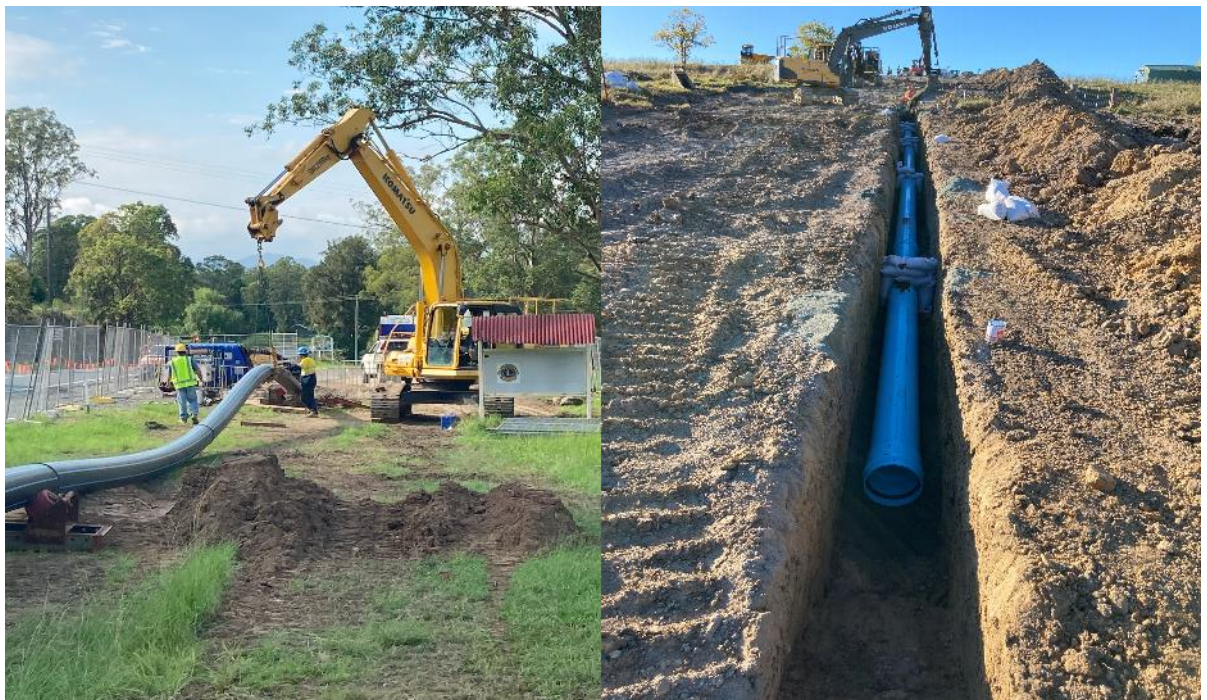
Figure 6: Laying of new rising main in Gloucester Water Supply System
