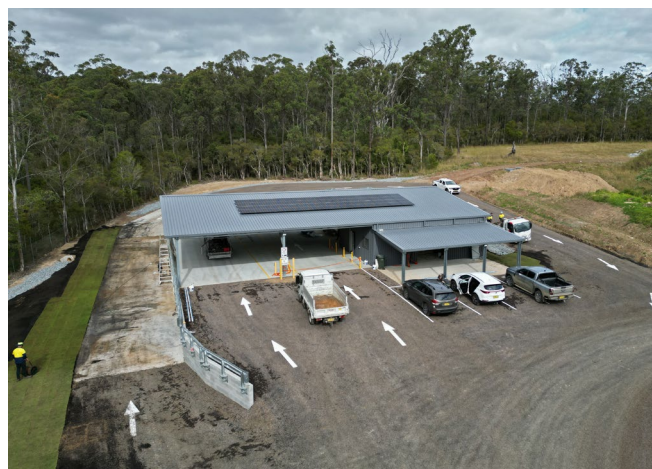
Stroud Waste Transfer Station
