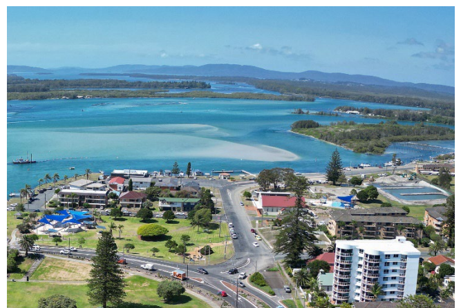
Dredging works near the Point Road boat ramp were completed.
