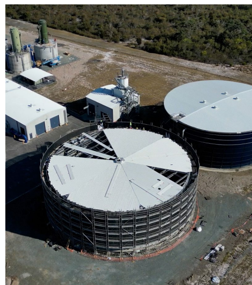
Nabiac Water Upgrade
