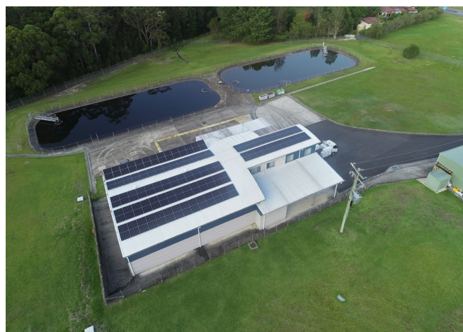
Solar Panels at Bulahdelah Water Treatment Plant
