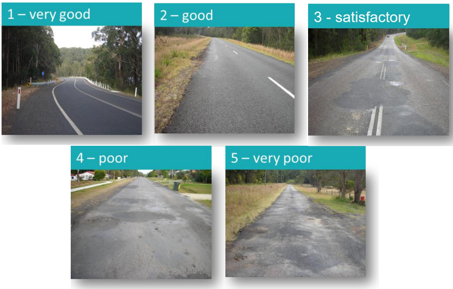
Figure 21 - Typical Examples of Condition Ratings
