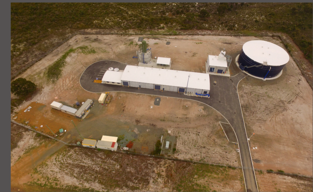
Top: treatment building. Below: aeration tower and pre-treatment tank.
