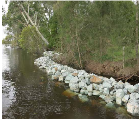
Figure 1.1.15 Rock fillets along the Wallamba River.
