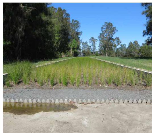
Figure 1.1.17 Pipers Bay Drive water quality garden.
