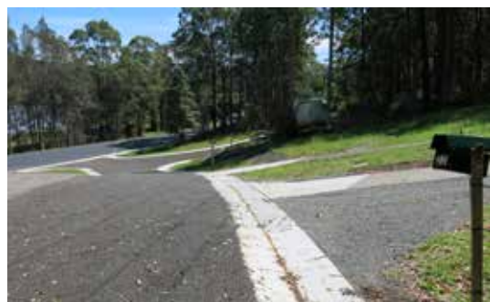
Figure 1.1.15 Gravel road sealing and table drain upgrade, Tarbuck Bay
