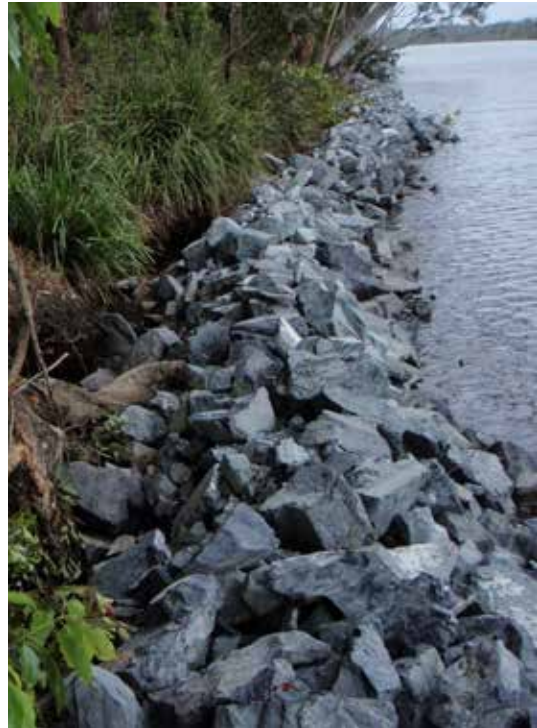
Figure 1.1.9 Erosion protection works on the Wallamba River
