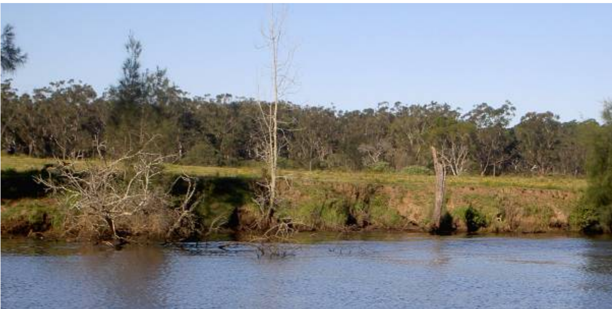
Figure 8: Slumping at ARL 21.5km.
