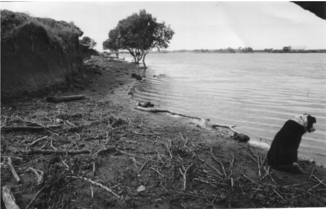
Figure 11: Project site pre-construction at Dumaresq Island in the Manning River, October 1999.
