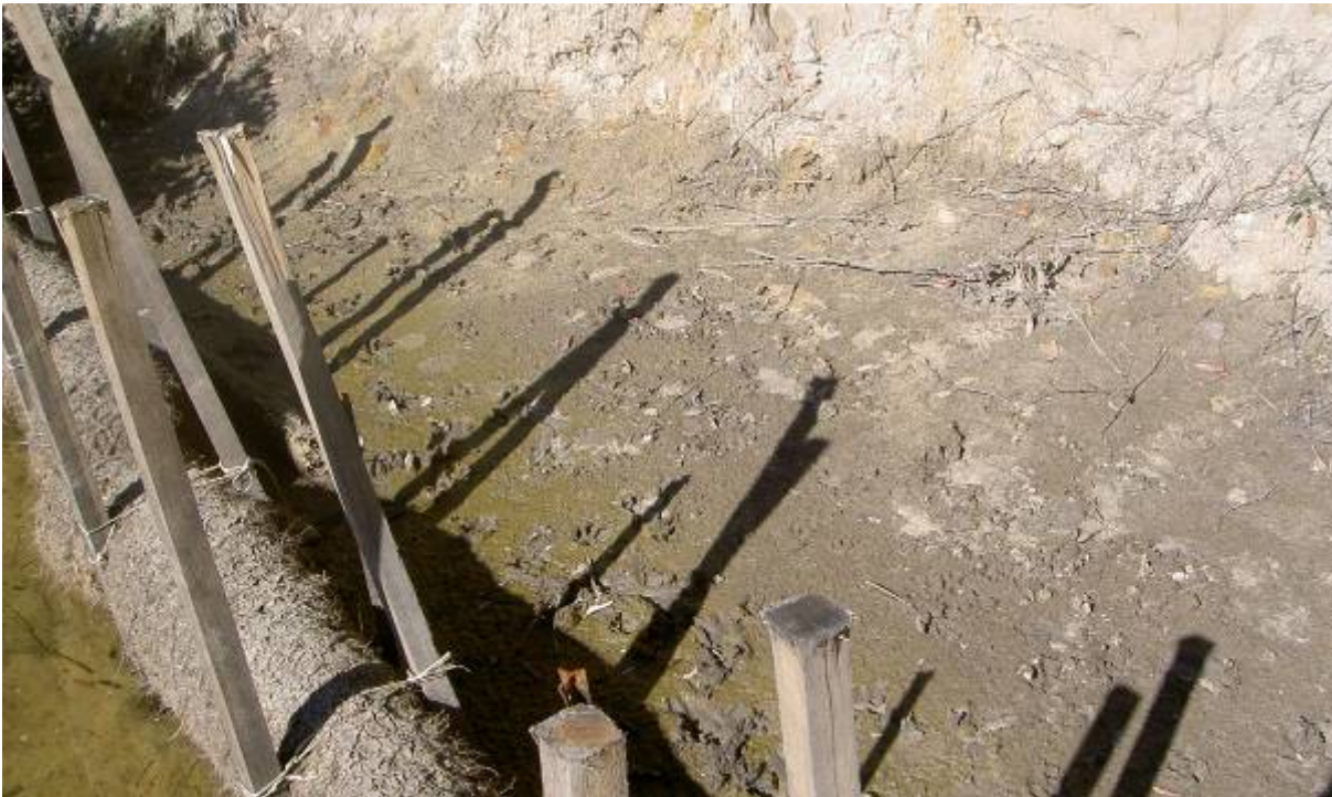
Figure 14: Sediment deposited behind recently constructed coir log walls, by May 2003 fresh.
