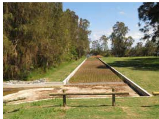
Figure 1.1.20 Pipers Bay Drive water quality garden (under construction)
