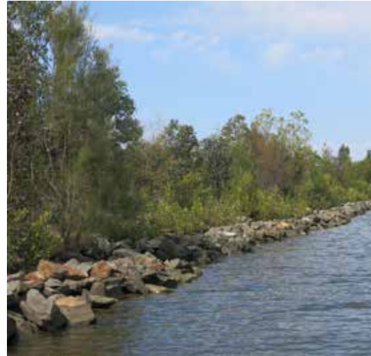
Figure 1.1.18 Rock fillets encourage the establishment of mangroves
