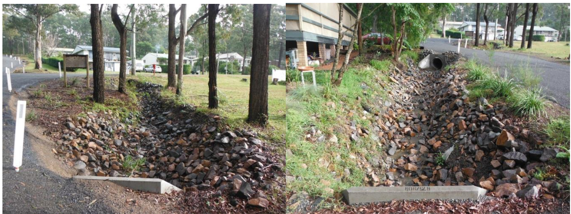
Figure 3-7 Upper and Middle Open Channel Reaches (looking upslope)
