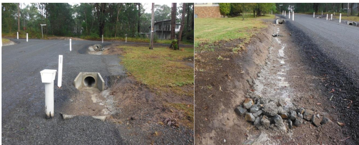
Figure 3-5 New Works in Upper Water Street
