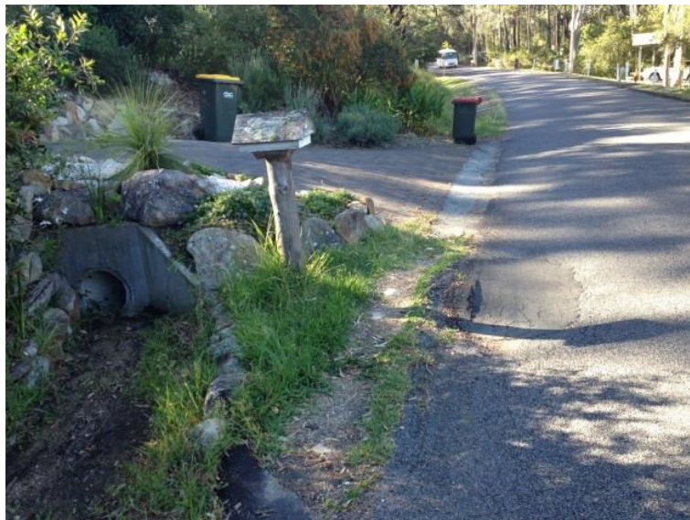
Figure 3-3 Example of Elevated Driveway Crossing
