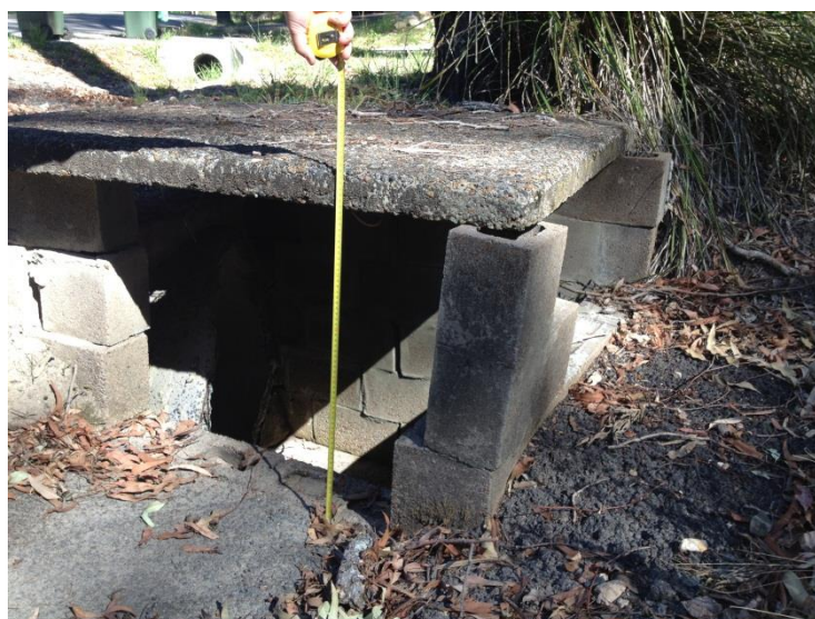
Figure 3-10 Drainage Inlet Opposite 70 Cove Boulevard
