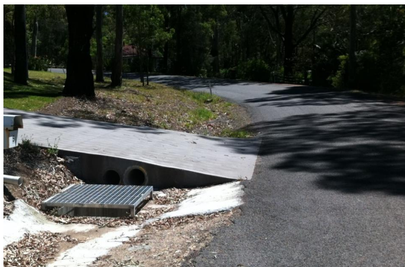
Figure 3-4 New Drainage Inlet Opposite 10 Cove Boulevard
