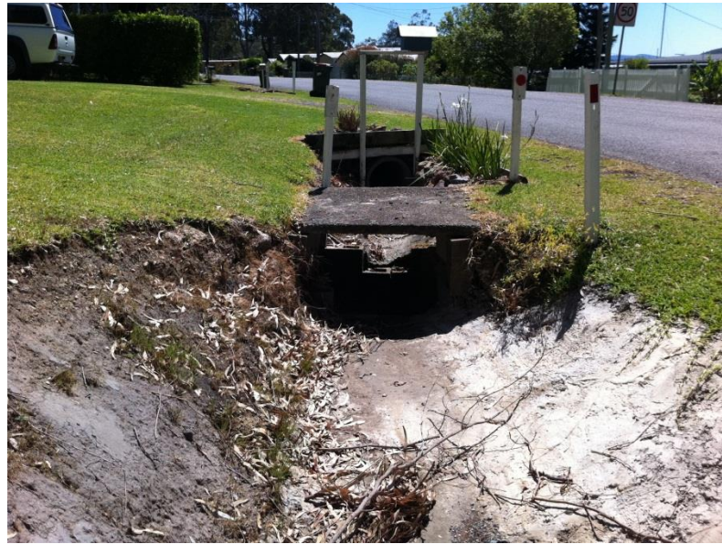
Figure 3-6 Drainage Inlet near Cove Boulevard / Water Street Intersection
