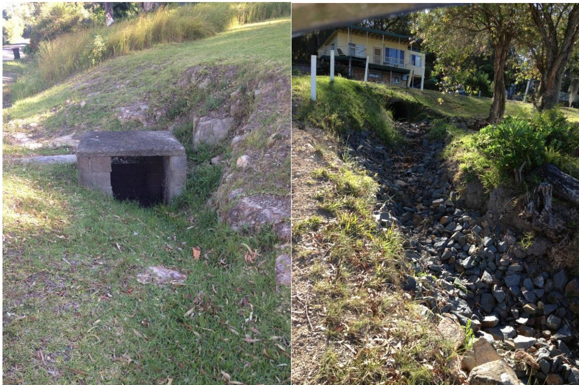
Figure 3-11 Drainage Inlet Opposite 108 Cove Boulevard and Rock Lined Channel
