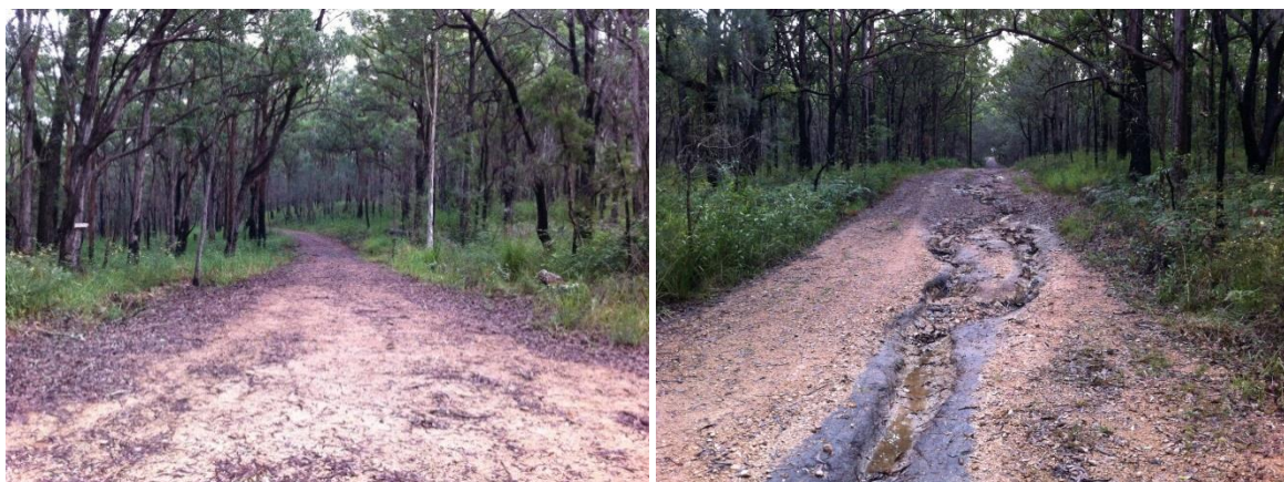
Figure 3-2 Unsealed Fire Trails - aligned along contours (L) and across contours (R)
