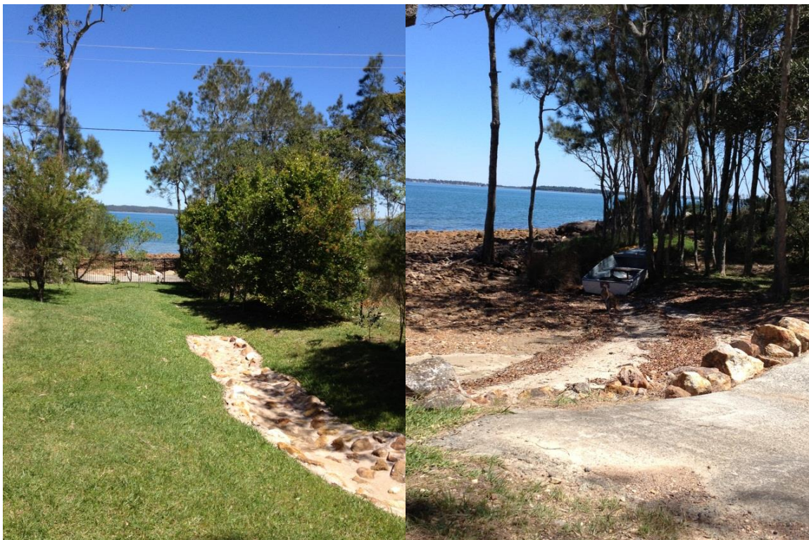
Figure 3-12 Existing Concrete Lined Overland Flowpath and Causeway at 33 The Esplanade
