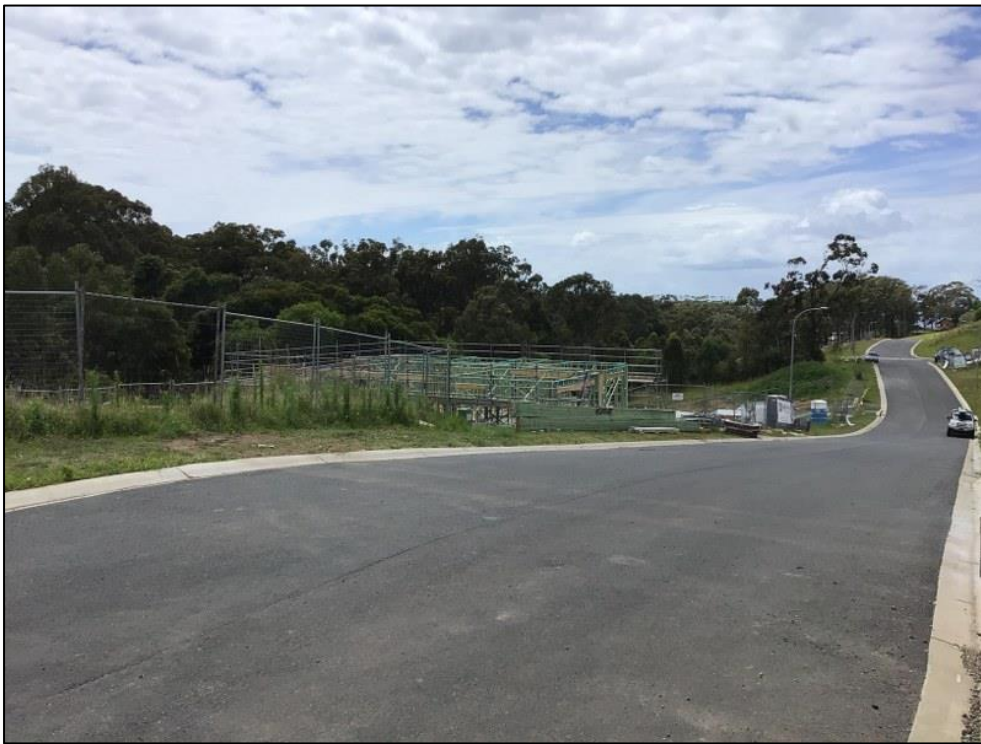
Plate 13 Residential development along Maslin Close
