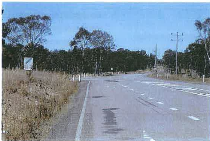
Main Entrance looking south
