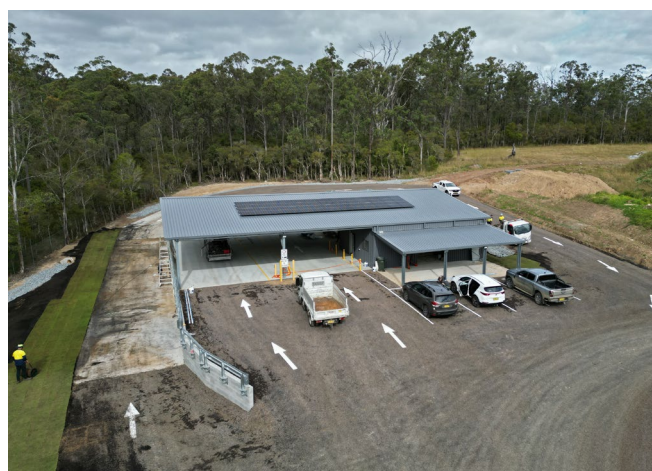
Stroud Waste Transfer Station
