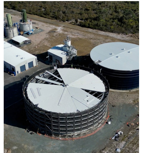
Nabiac Water Upgrade
