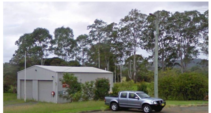
Additions will be made to the Wallaby Joe Rural Fire Station in Wingham
