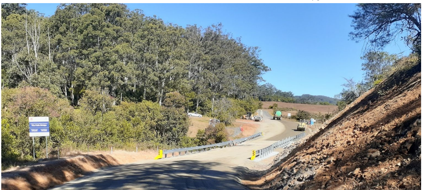
The Falls Bridge, Elands
