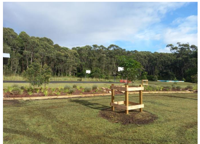
Beautification works completed at Smiths Lake Recreation Area.
