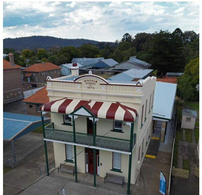
Libraries: Façade makeover for the Wingham Library.
