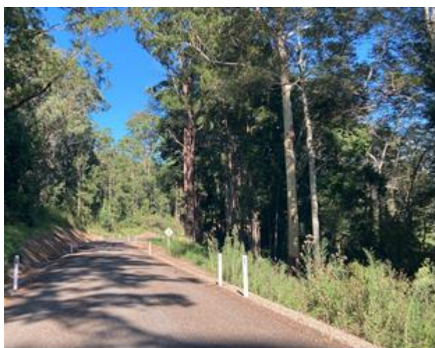
Hannam Vale Road & Waitui Road, Hannam Vale & Waitui as part of the $7.5 million Local Roads Program
