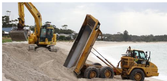
Jimmys Beach: 20,000 cubic metres of sand per year is moved onto the beach to warn off erosion.
