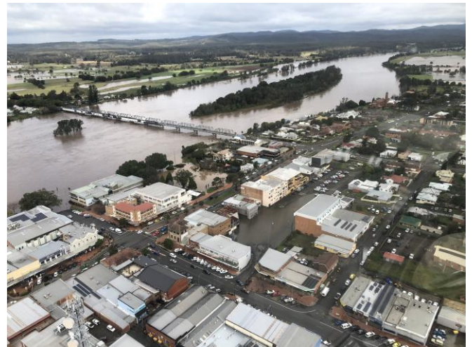
Taree inundated by flood waters during the July 2022 flood event that affected our major centres and several townships within our local government area.
