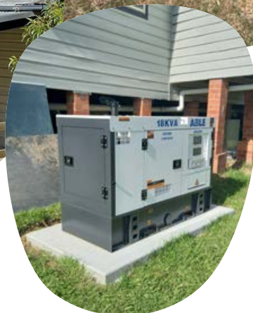
Right: New generator installed at Moorall Creek
