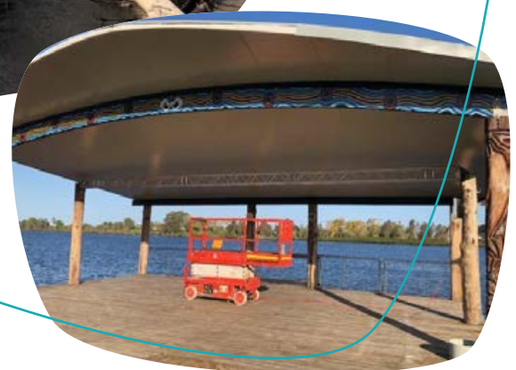
Flood rectification works at the River Stage in Taree
