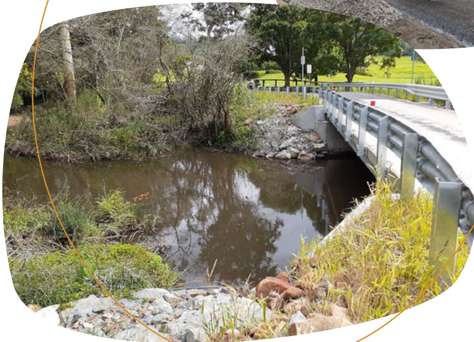
Top: Cox Bridge Caparra Road, Wherrol Flat
