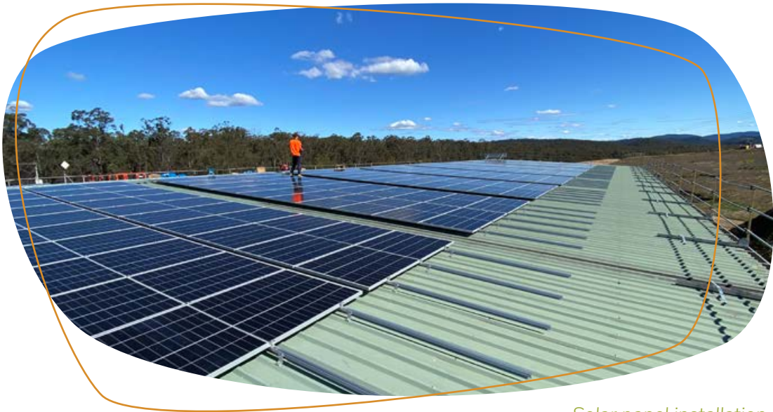
Solar panel installation at the Taree Landfill transfer station
