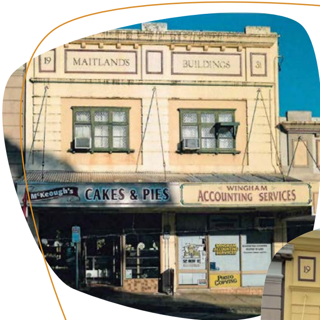
Maitland Building in Wingham before and after painting and repairs
