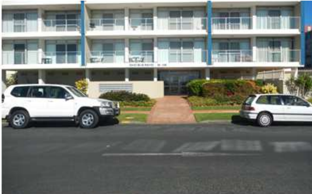
Image 1- Existing Access to "Oceanic"
