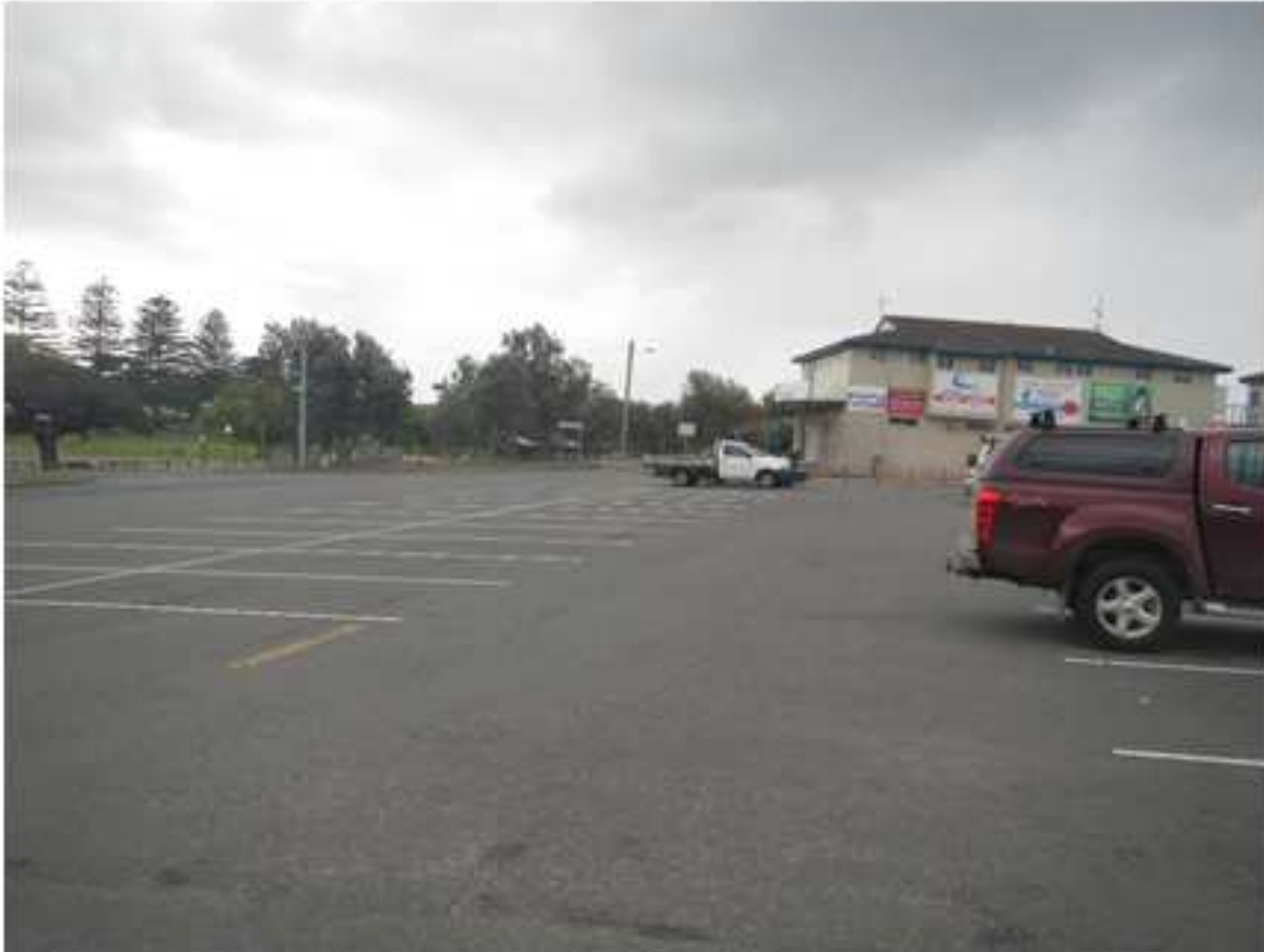
Image - Bennetts Beach Car Park Existing Linemarking
