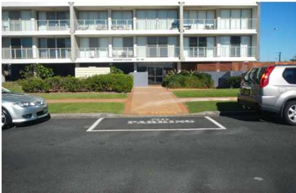
Image 2- Existing "No Parking" pavement marking at the Access to 2-6 North Street
