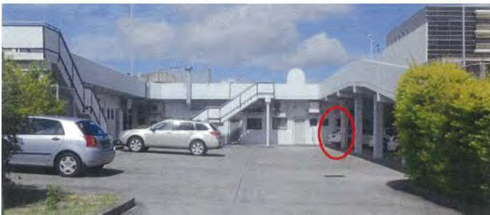
Figure 3 Existing car parking showing car parking below roof overhang
