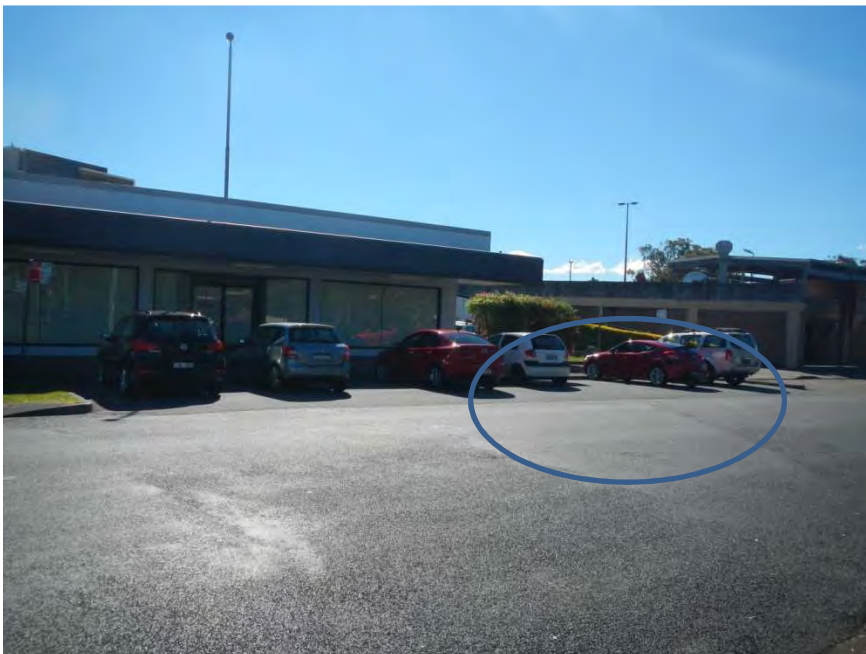
Image: Location of proposed dedicated parking bays on Parkes Street (date taken 19/10/16)
