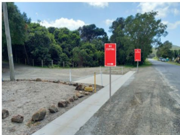
Near eastern driveway
