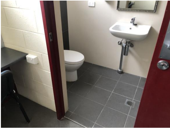
Typical dressing room WC
