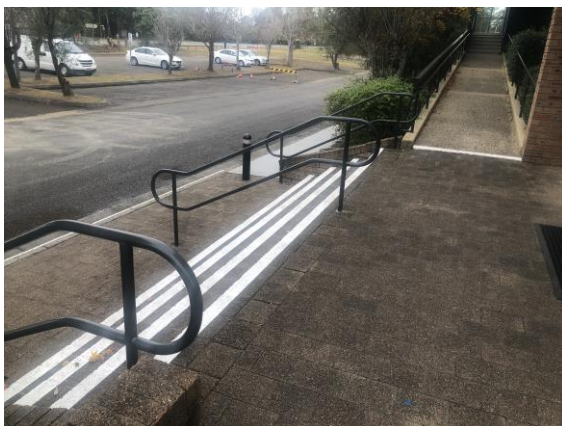
East entry steps
