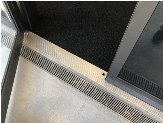
Entry flush drain
