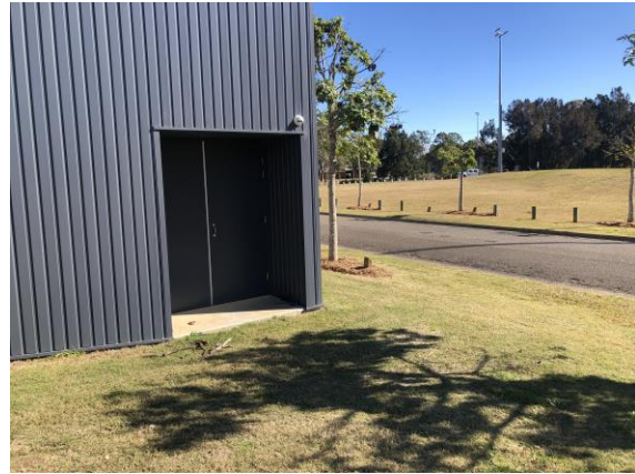
NW stair exit
