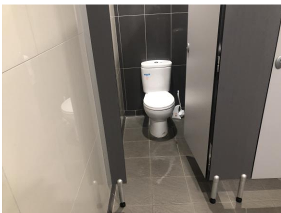
Typical WC cubicle
