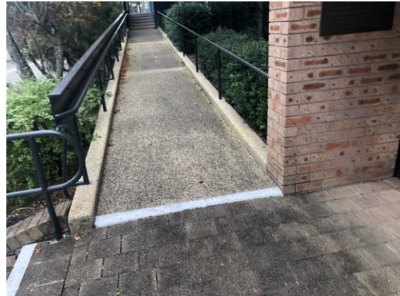
East external ramp
