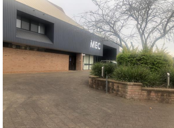
MEC north walkway approach
