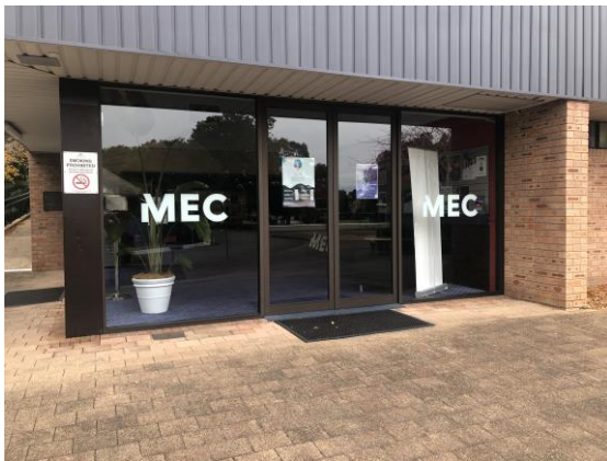
MEC north entry
