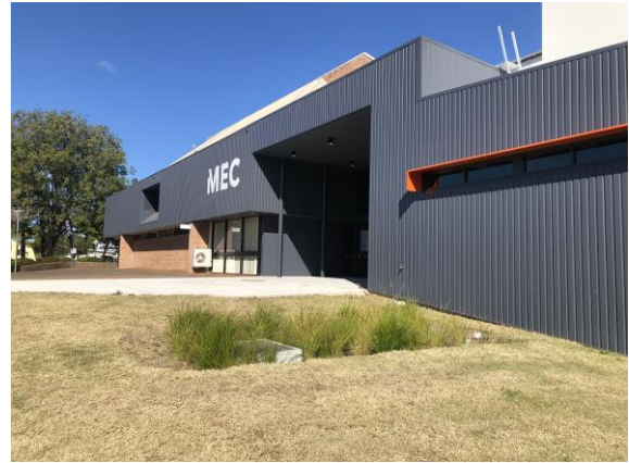
West entry rain garden
