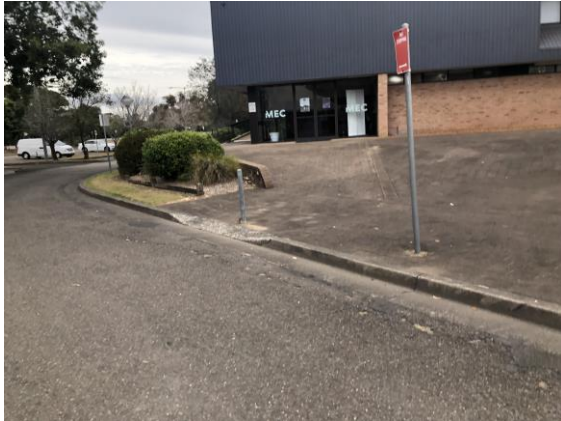
MEC north kerb ramp
