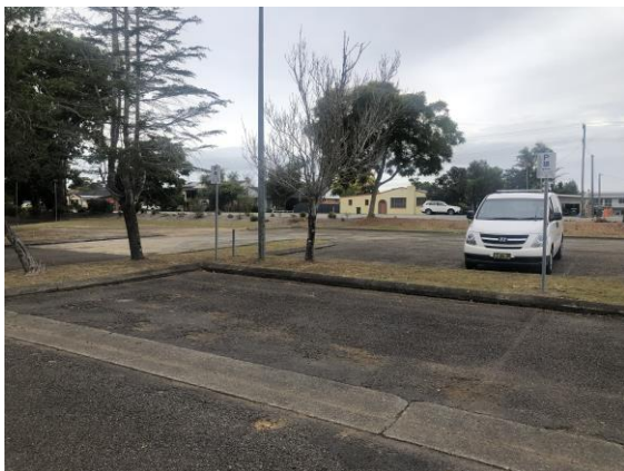
Non-complying accessible parking
