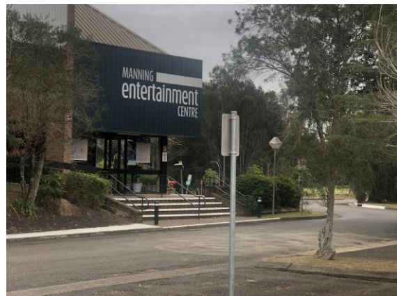
MEC east entry steps
