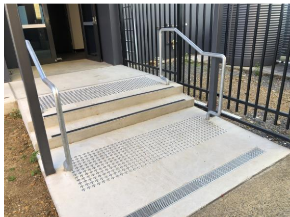
Steps between Studio and MEC
