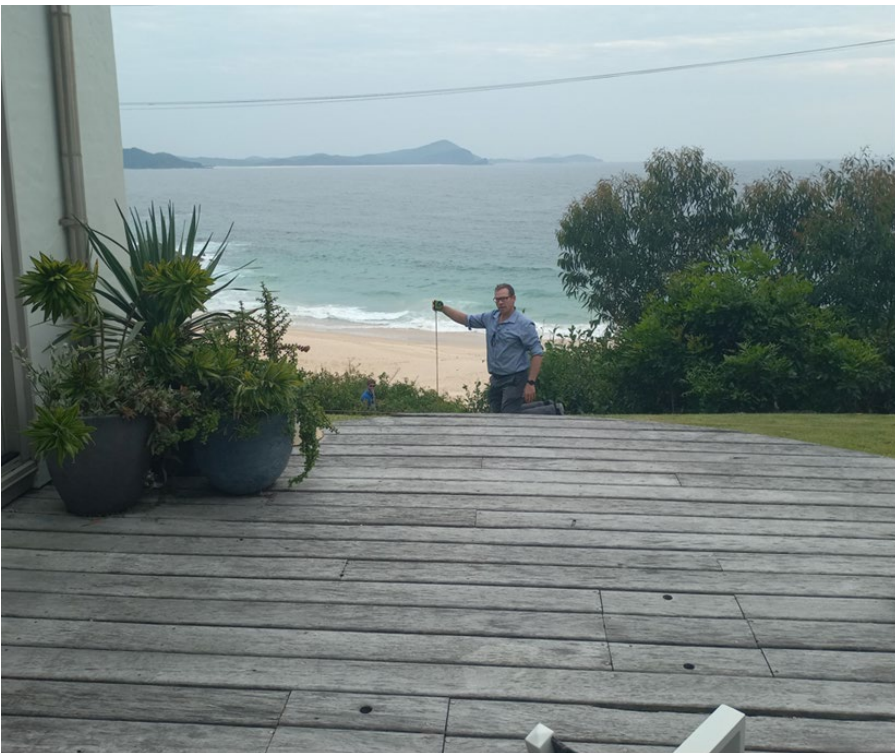
Figure 29 - View from the lower ground floor deck. The tape measure illustrates the height of the safety rail. (Source – Council staff inspection).
