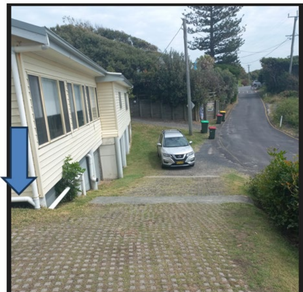
Figure 31 - shows the front of 10 Kinka Road. Photos were taken standing in front of the eastern most, northern windows, which was a living/dining area.
