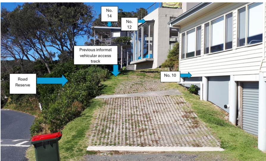
Figure 6 – Locality photo showing relationship of adjoining properties, previous access track and road reserve (Mid-Coast Council)
