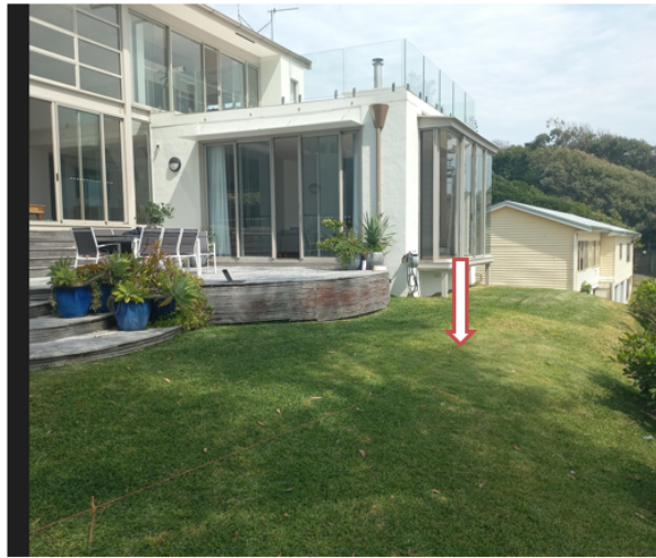
Figure 10 - Arrow shows the location of string line showing front boundary, where safety rail/retaining wall will be located.
