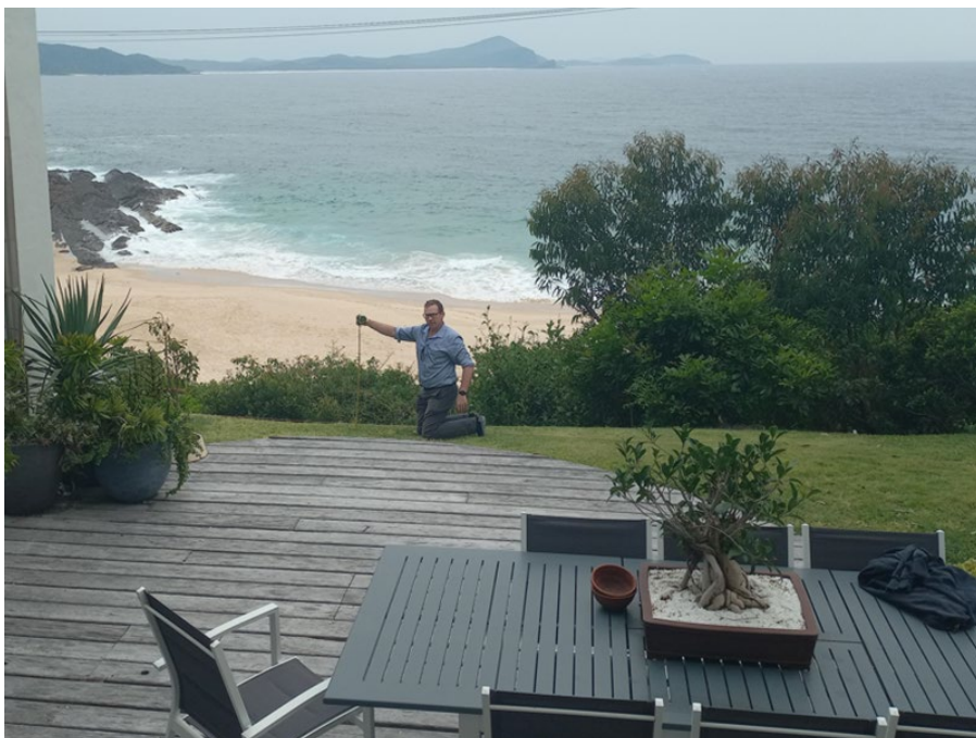
Figure 27 - View from the raised section of the living area ground floor. The tape measure illustrates the height and approximate location of the safety rail. (Source – Council staff inspection).
