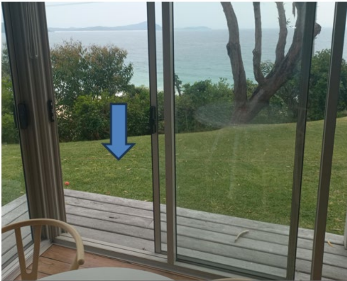
Figure 30 - View from the lower ground floor eastern side living area. The safety rail finishes at the approximate location of the arrow, therefore with the existing vegetation the barrier will pose minimal impact on the view . (Source – Council staff inspection).
