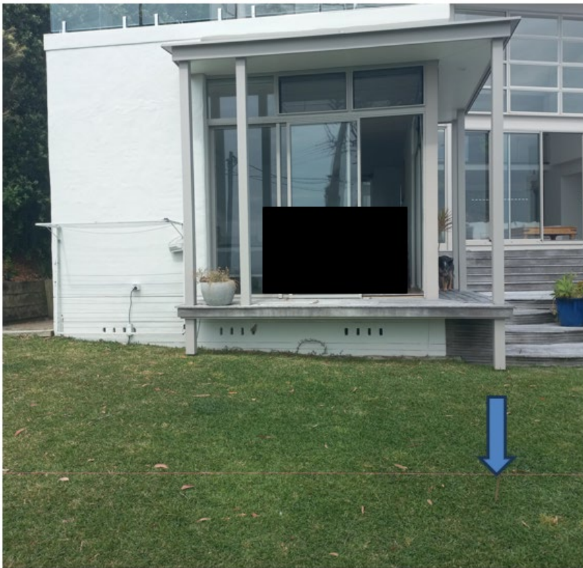
Figure 20 illustrates the blue arrow where the safety rail ends and the car will be closer to ground level height.
