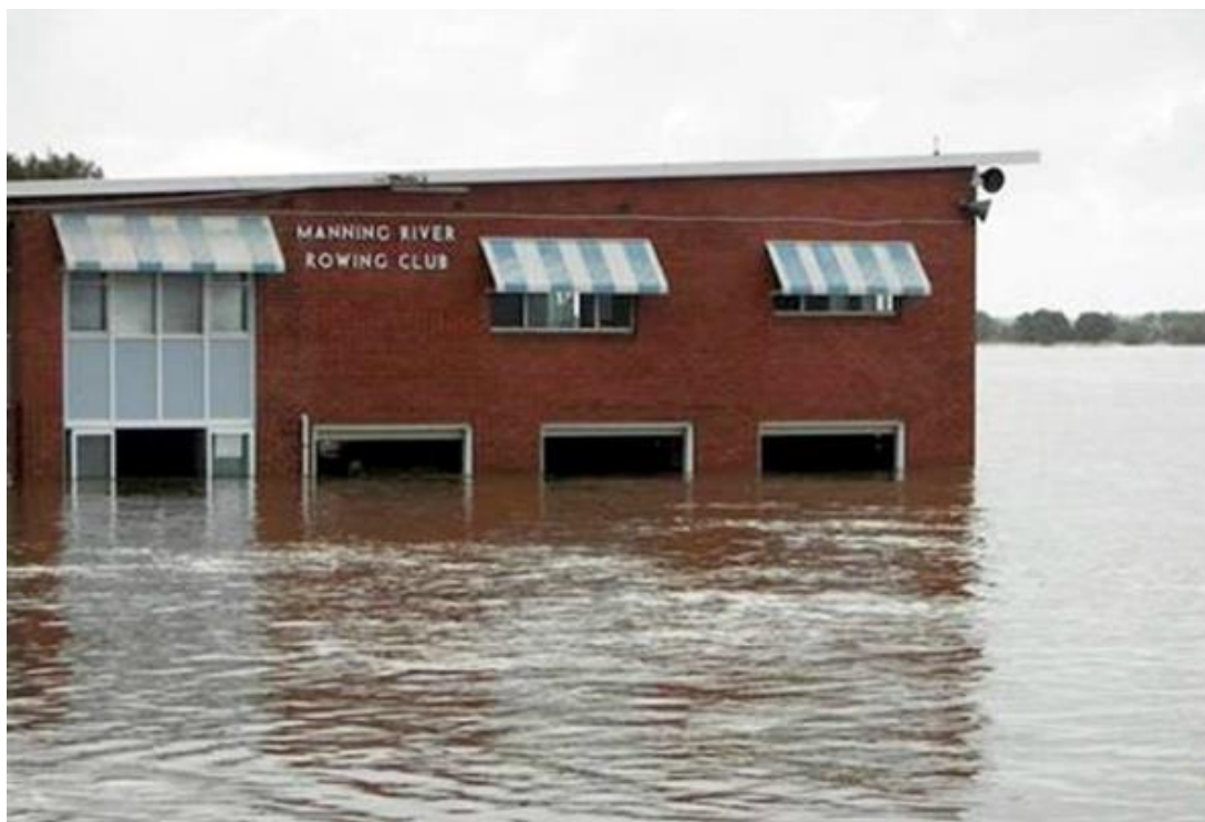
Figure 2-7 June 2011 Flood - Manning River Rowing Club, Taree
