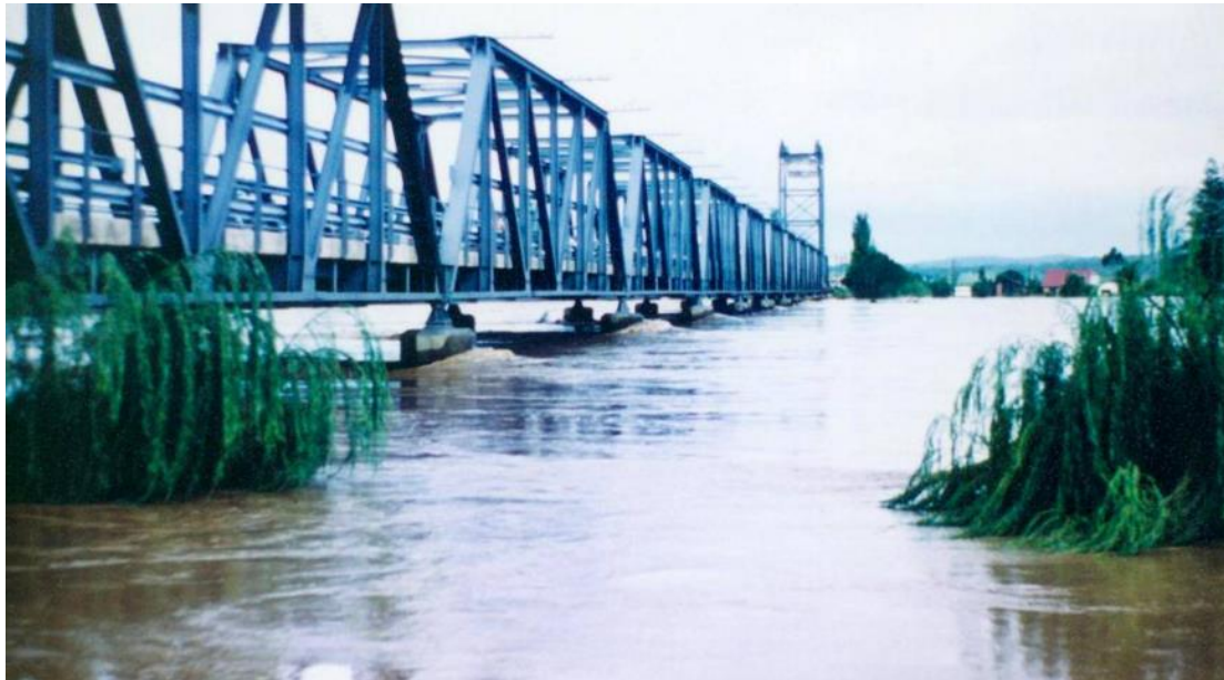
Figure 2-2 March 1978 Flood - Martin Bridge, Taree
