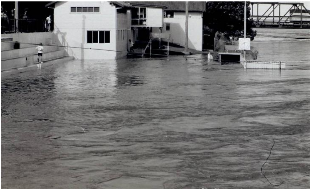
Figure 2-5 February 1990 Flood - Former Swimming Pool, River Street, Taree
