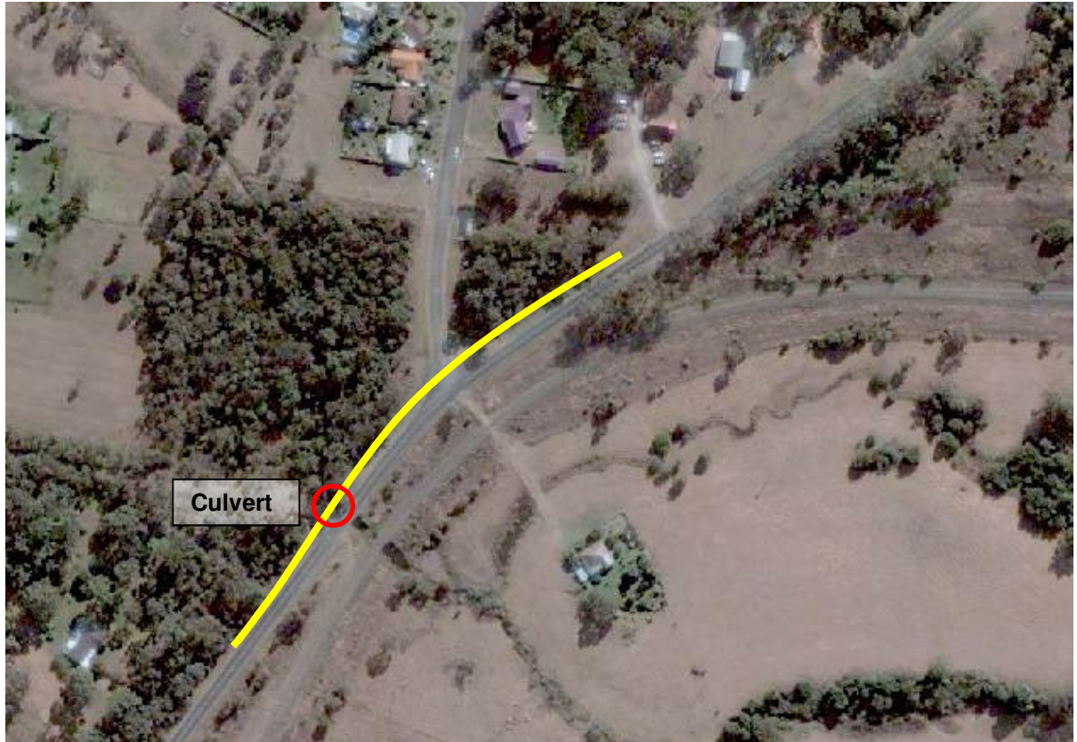
Figure 12: Location of proposed upgrade by raising the stretch of road along Cundle Road, Lansdowne
