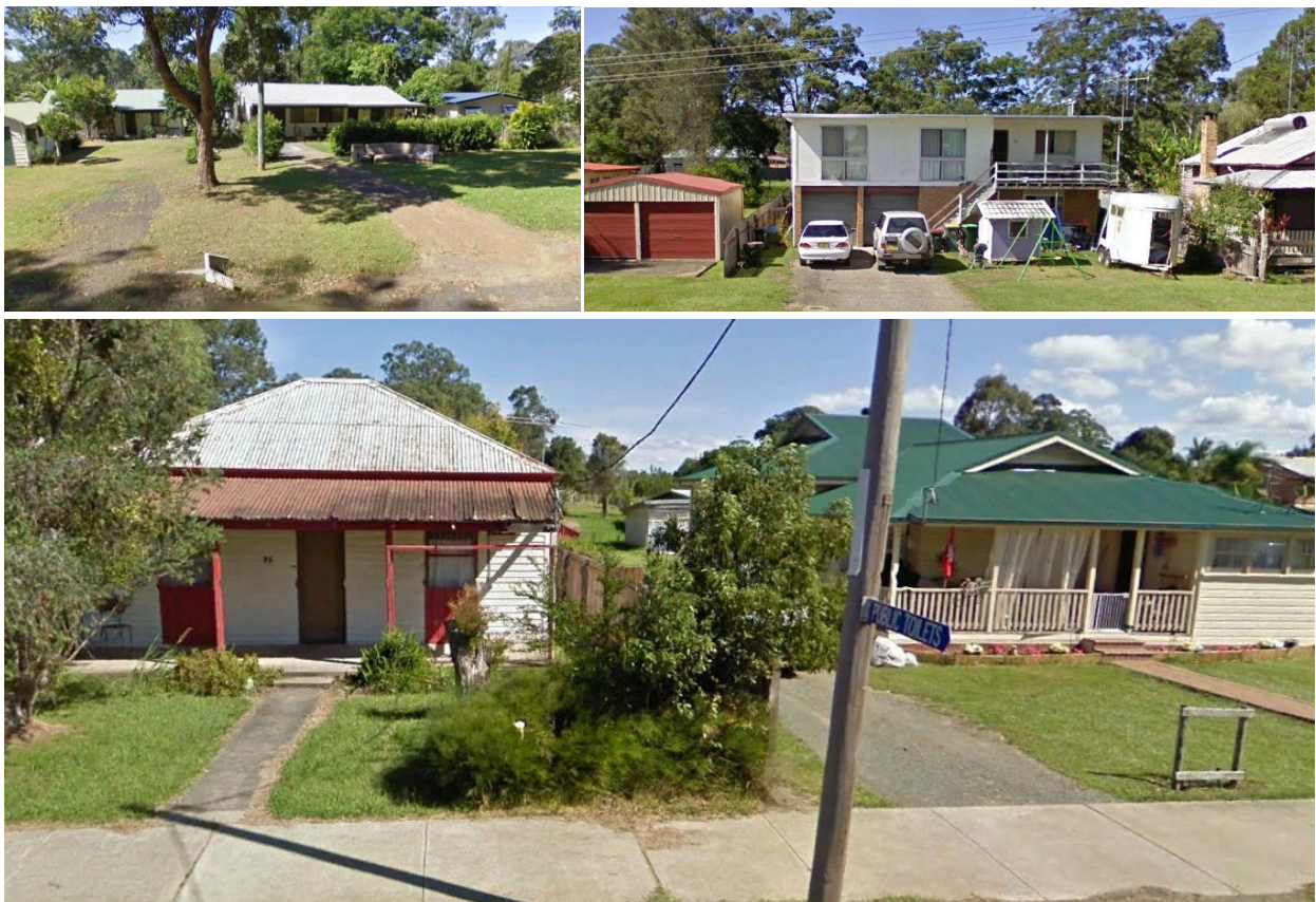
Photograph 18: Examples of houses without significant clearance of the ground floor level above surrounding areas
