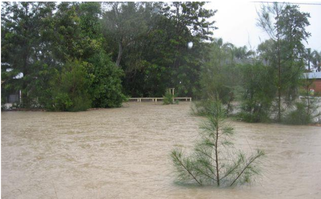
Photograph 6: Flooding of Nabiac Street footbridge in June 2007 (source: Bruce Weller)
