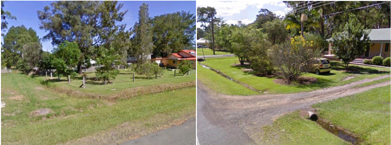
Photograph 2: Roadside drainage swale on Nabiac Street (left) and Hoskins Street (right)
