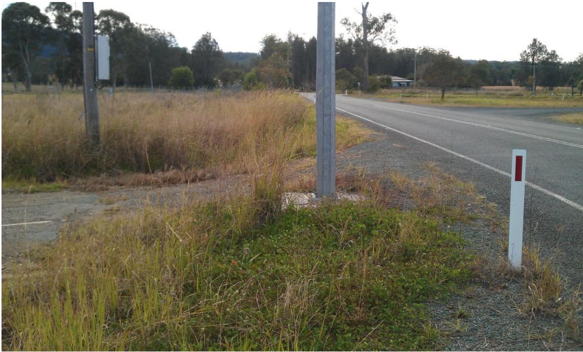
Photograph 16: The re-grading of Candoormakh Creek Road (at right) is significantly higher than the previous Wallanbah Road levels (at left)
