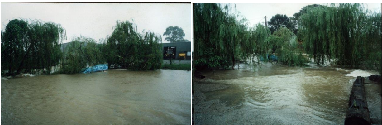
Photograph 8: “Industrial culverts” at Ferris Place blocked during February 2002 flood event. From east (left) and west (right).
