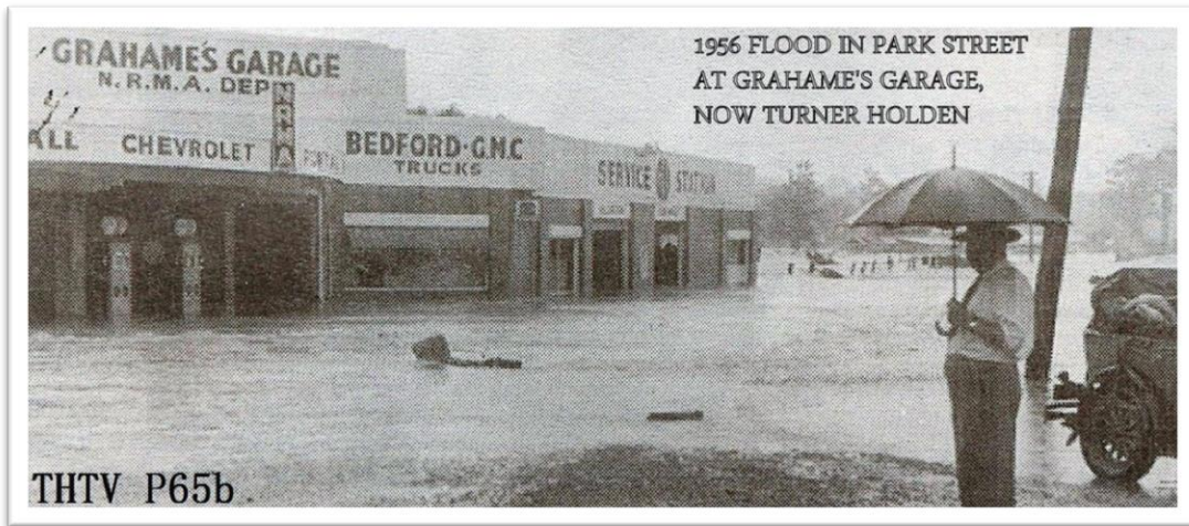
Figure 2-5 Grahame's Garage during the 1956 Flood Looking NW along Park Street
