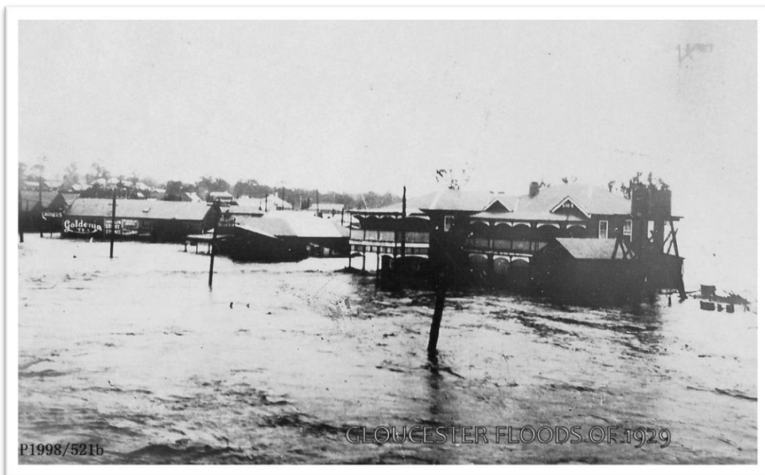
Figure 2-2 Royal Hotel during the 1929 Flood Looking South Along Church Street
