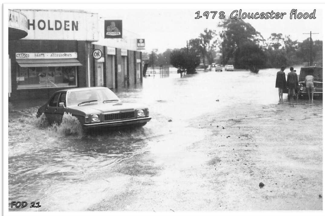
Figure 2-13 Holden Garage during the 1978 Flood Looking NW along Park Street
