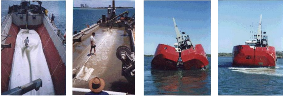
Figure 2.15: Placement of a Geotextile Tube by dropping from a Split-Hull Vessel (Photos: ICM)
