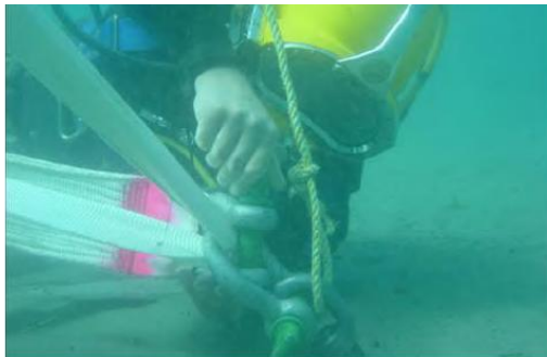
Securing Reef Panel to Seabed Anchor
