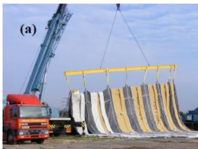
Figure 2.16: RAD Reef Construction Method at Mount Maunganui (ASR, 2008a)
