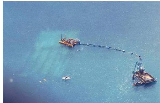
Filling Geotextile Tubes
