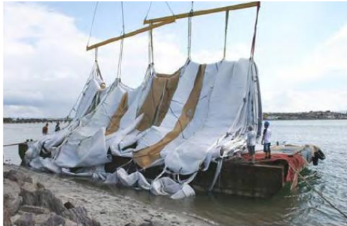
Loading Reef Panel onto Barge
