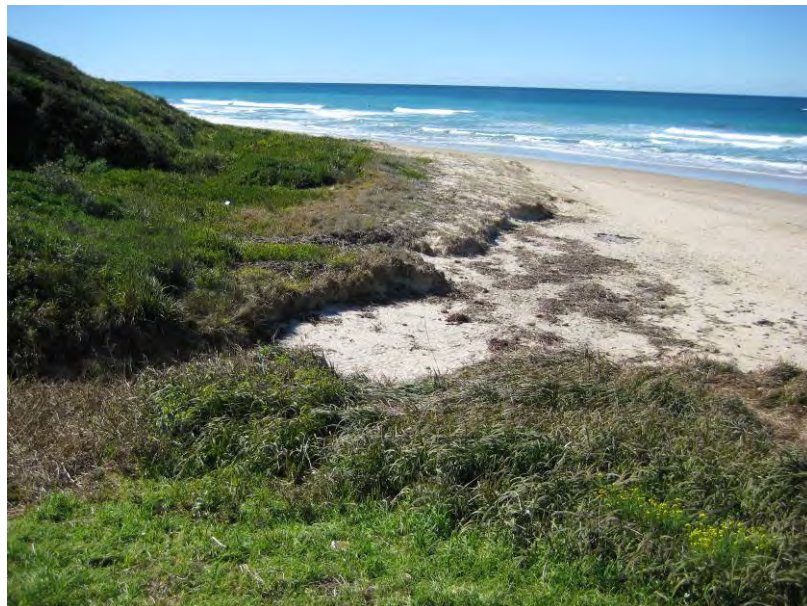
Plate 14 – Old Bar Beach erosion caused by the stormwater drain
