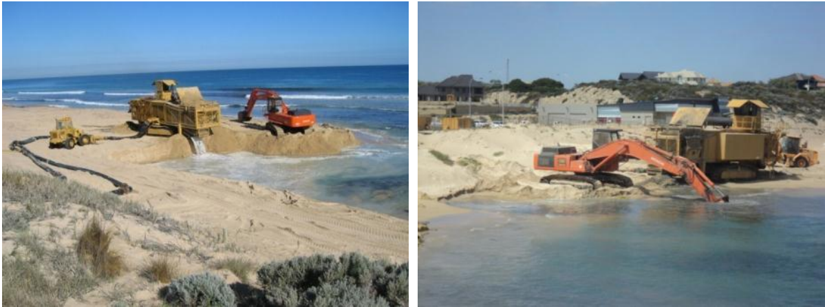
Figure 2-4 A tracked mobile pumping unit operating in Dawesville, Western Australia.
