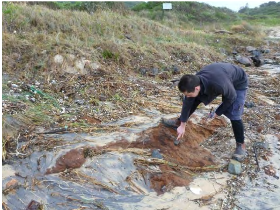
Figure 4-7 Indurated Silty Sands with Gravels Exposed at the Base of Southern Blueys Beach.
