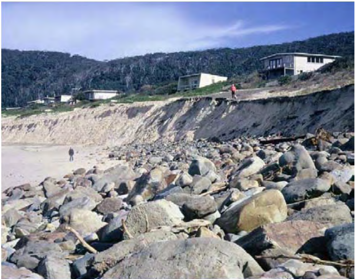
Figure 4-5 Exposed Boulder Beach at Northern Blueys Beach, Following a Severe Storm in May 1974 (Source: WorleyParsons, 2011)
