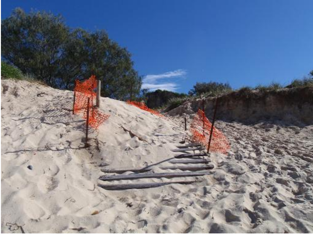
Figure 31: Damaged board and chain access to One Mile Beach (July 2010)
