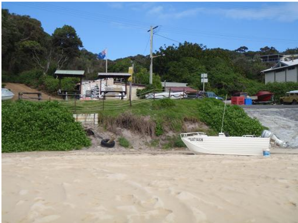
Figure 50: Erosion along Boat Beach and ad hoc protection (July 2010)
