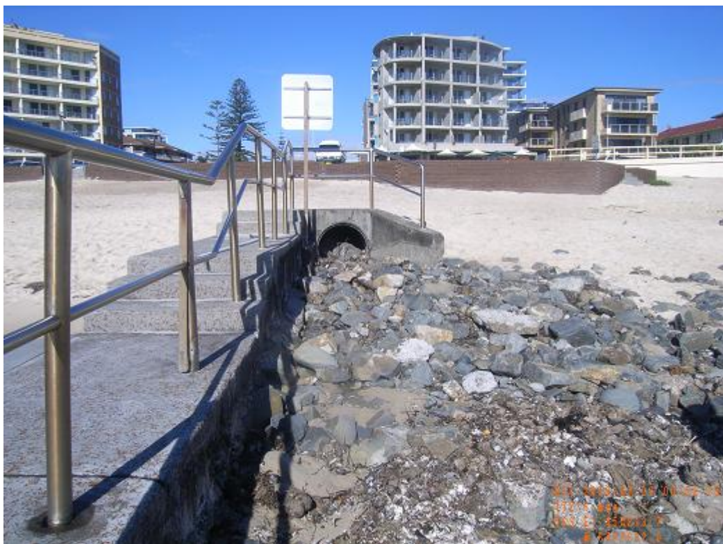
Figure 22: Stormwater outlet adjacent Main Beach swimming pool (July 2010)
