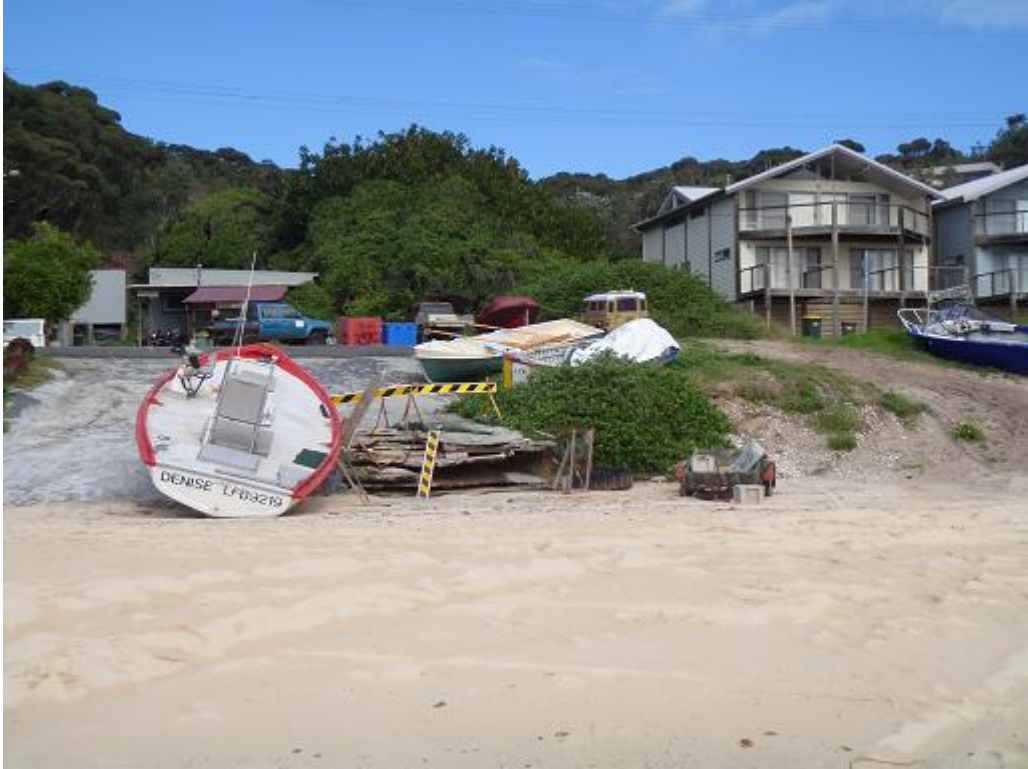
Figure 51: Damaged private boat ramp at Boat Beach (July 2010)
