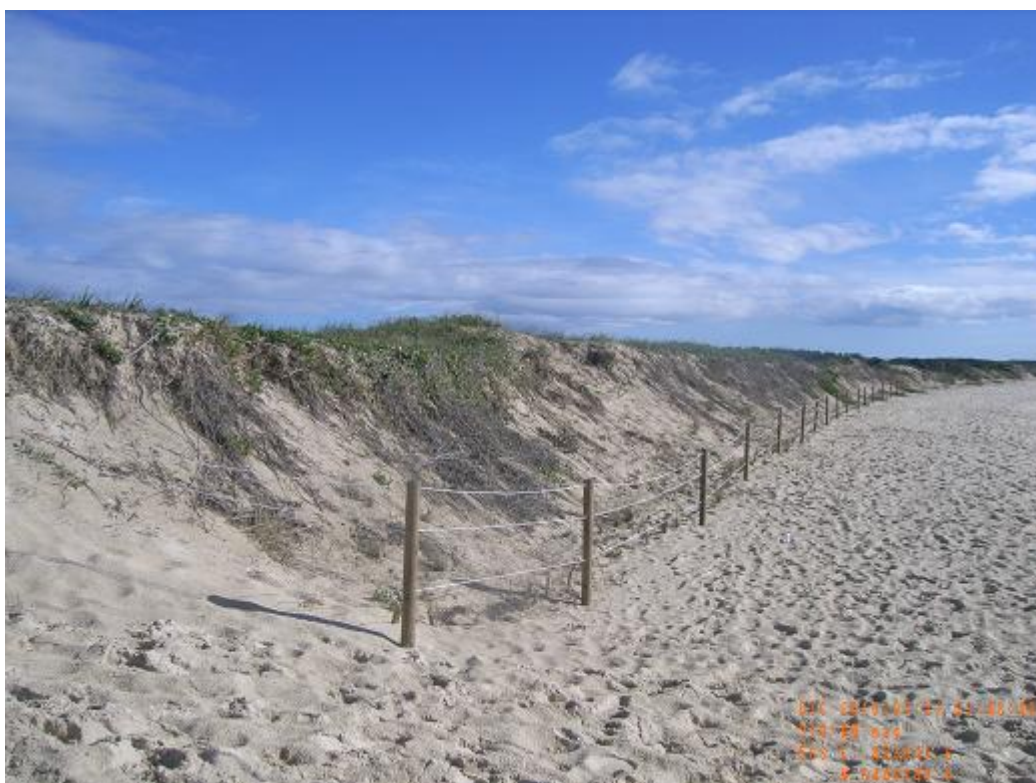
Figure 14: Storm bite behind the fences at the southern end of Nine Mile Beach (July 2010)
