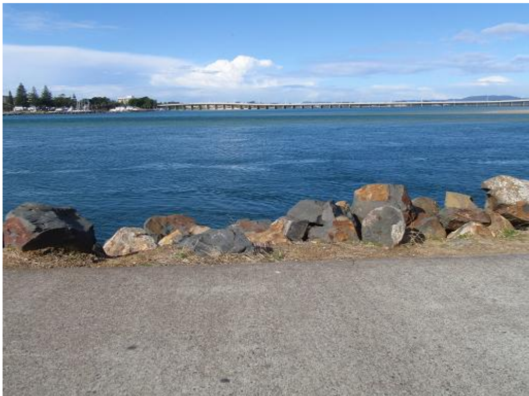
Figure 12: Seawall within Wallis Lake entrance (July 2010)
