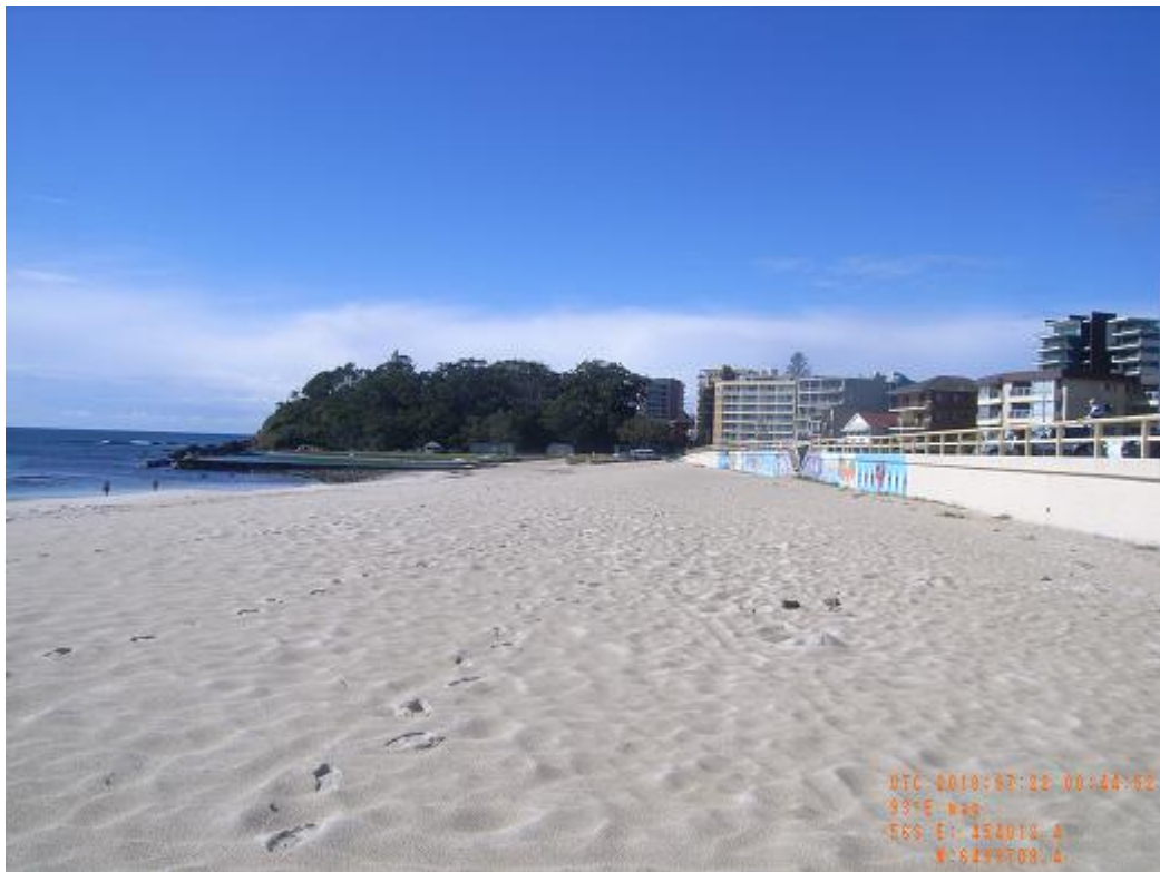
Figure 19: Vertical seawall at Main Beach (July 2010)
