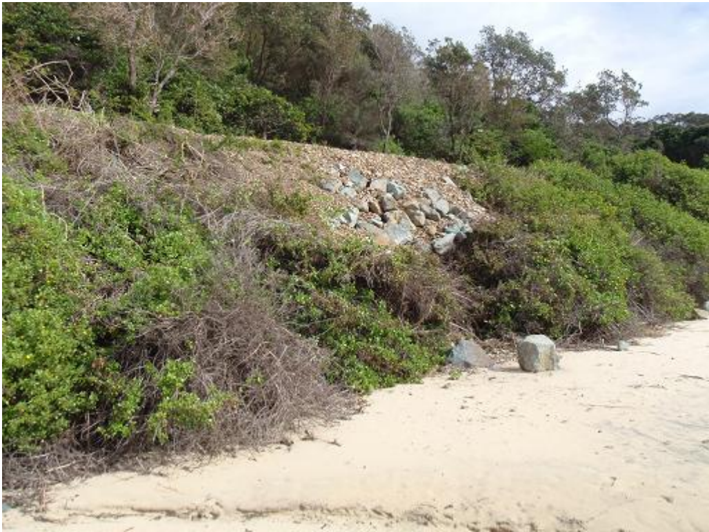
Figure 47: Dumped rocks to protect Seal Rocks Road at Number One Beach (July 2010)
