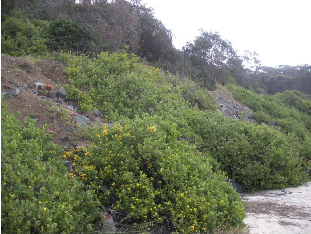
Photo 3: View of the slope failures along Number One Beach.
