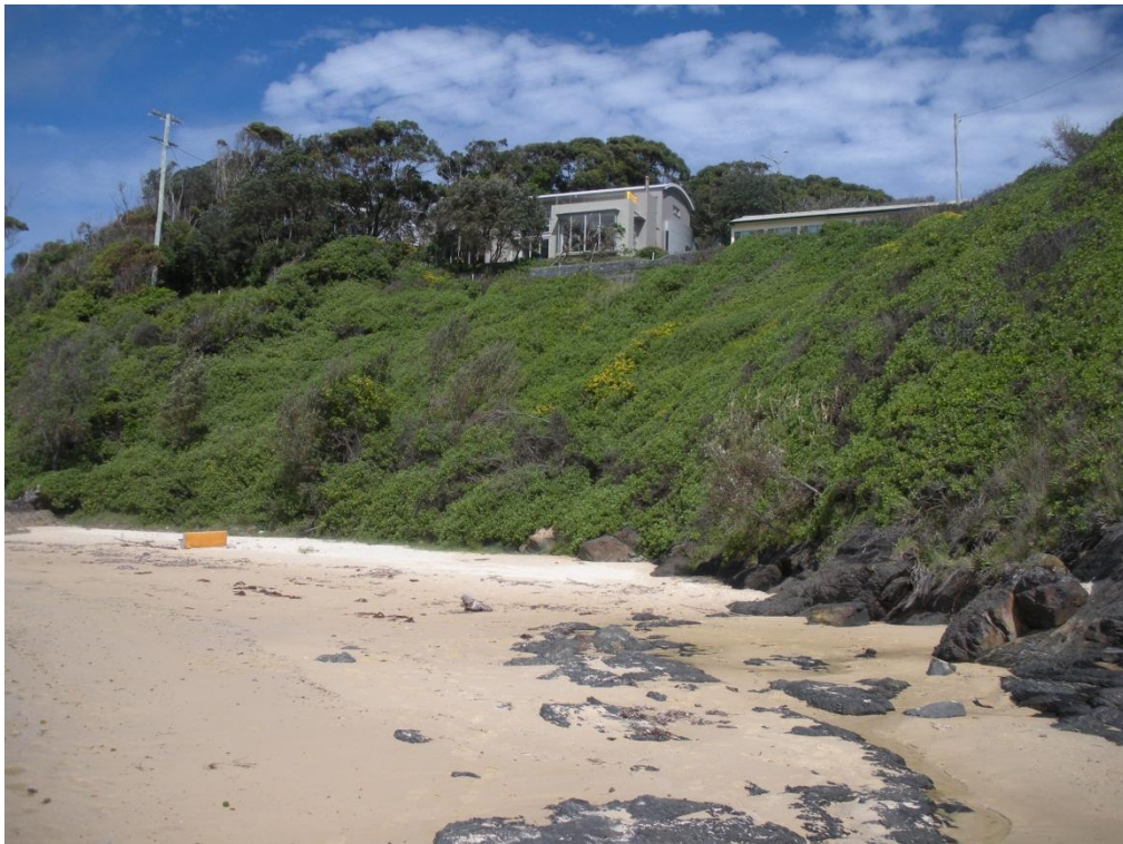
Photo 1: View of the area inspected on Boat Beach including the gabion wall at the crest of the slope.
