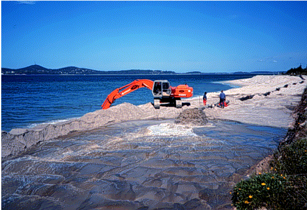
Figure 33: Beach Nourishment construction, Jimmy's Beach Port Stephens
