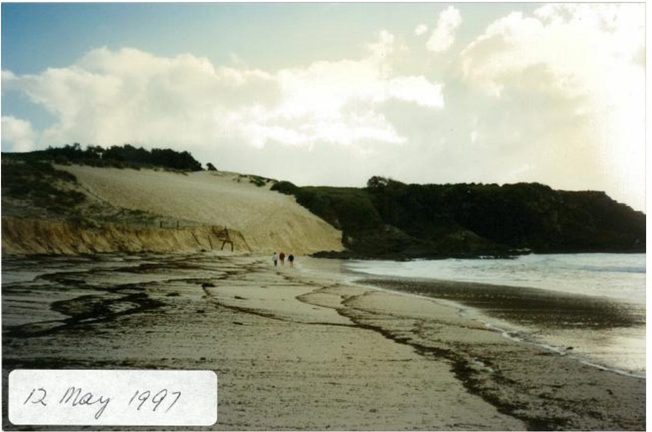
Figure A.5: Erosion generated by May 1997 storm event, One Mile Beach (courtesy Great Lakes Council)
