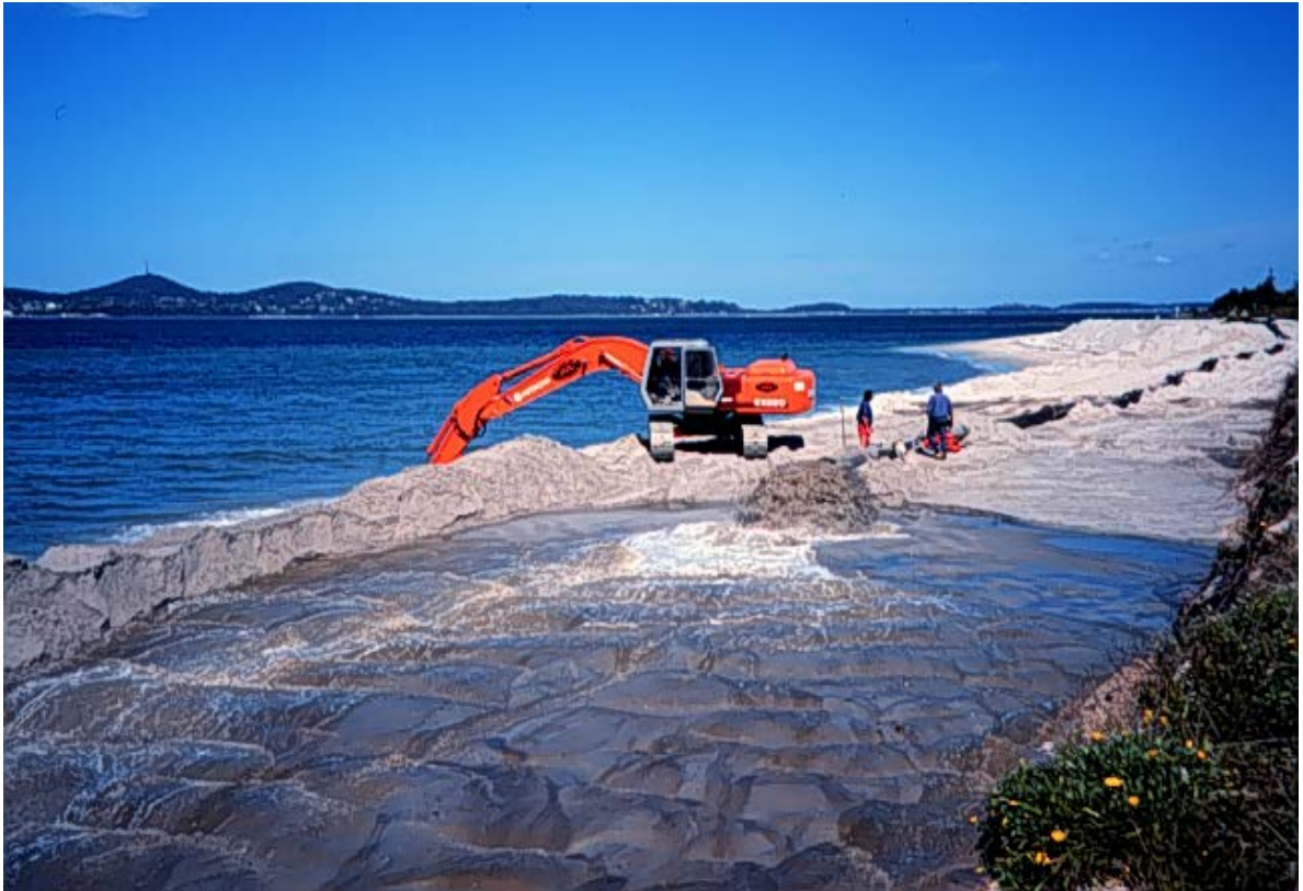
Figure 1 Beach Nourishment works at Jimmys Beach
