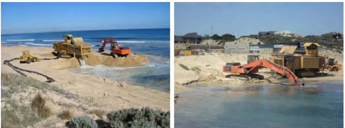
Figure 3 Tracked mobile hopper pumping unit operating in Dawesville, Western Australia
