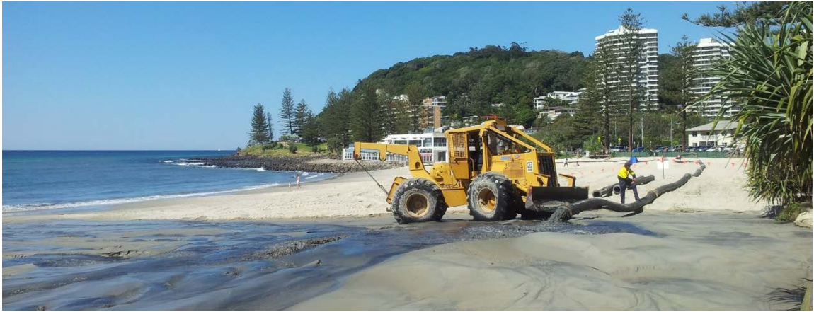
Figure 2 Sand being pumped onto beach Burleigh, Queensland Australia
