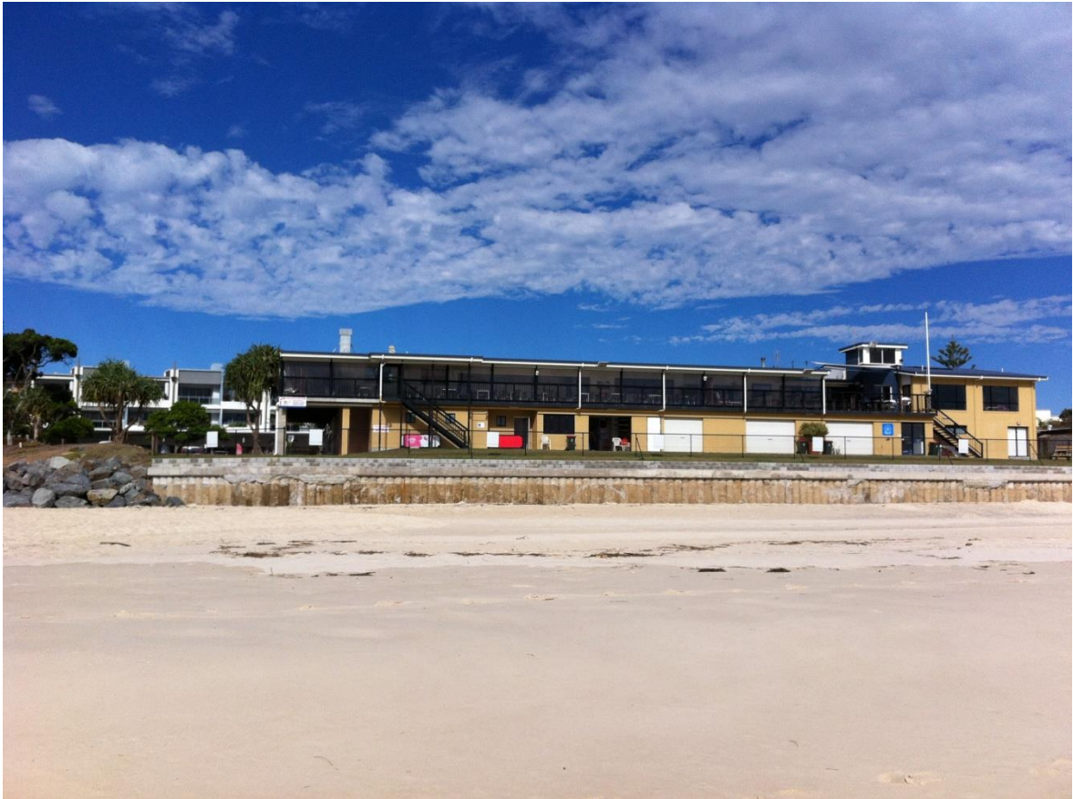
Figure 6 Cudgen Headland SLSC Seawall, Kingscliff Beach, northern NSW
