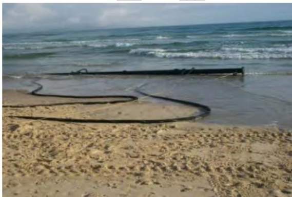
Figure 5 The Noosa trial Sand Shifter unit sourcing sand from the shore (left) and onshore booster pumps and pipework (right)
